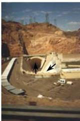
Arrows show the flow that would come over the spillway into a collection channel and then flow into a tunnel. The flow in the collection channel during a flood is unsteady and nonuniform but more specifically is unsteady, spatially-varied flow because the discharge is changing in the flow direction.
